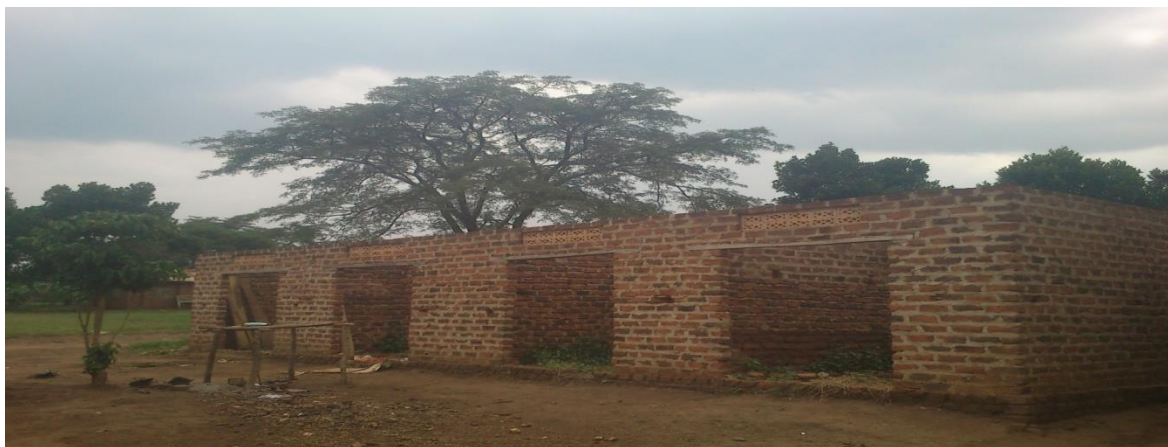
A front view of the site where construction had started.
