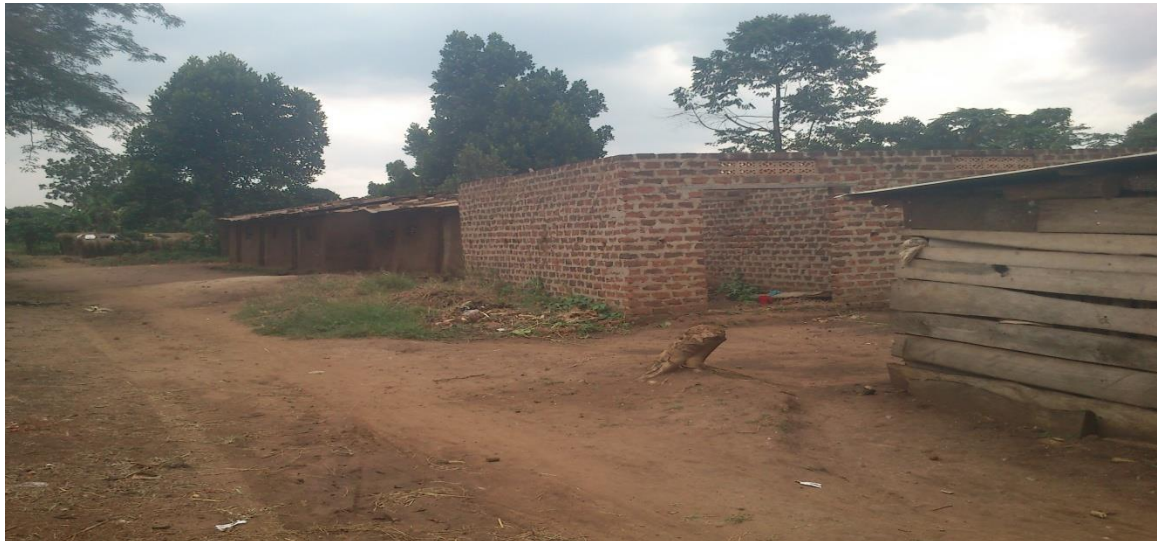
Aside view of the structures which were under construction
